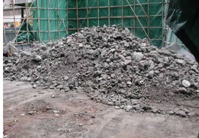
Figure 122 Sorted broken concrete (Source: Civil Engineering & Development Department)
