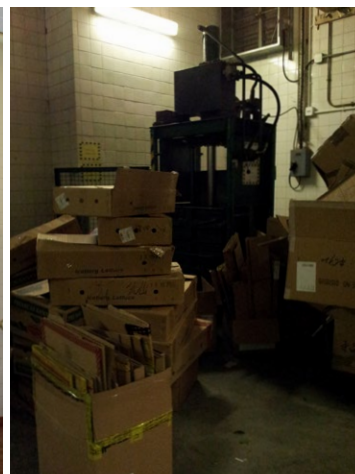
Figure 147 Baler for compacting recyclable (Source: Swire Properties Limited)
