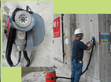
Figure 136 Grinding machine attached to a vacuum cleaner (Source: Environmental Protection Department)
