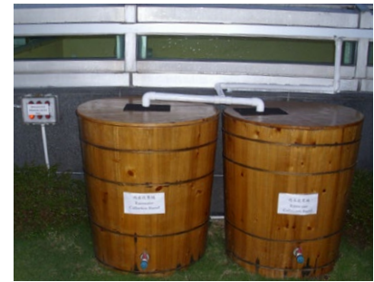
Figure 110 Simple rainwater harvesting system
