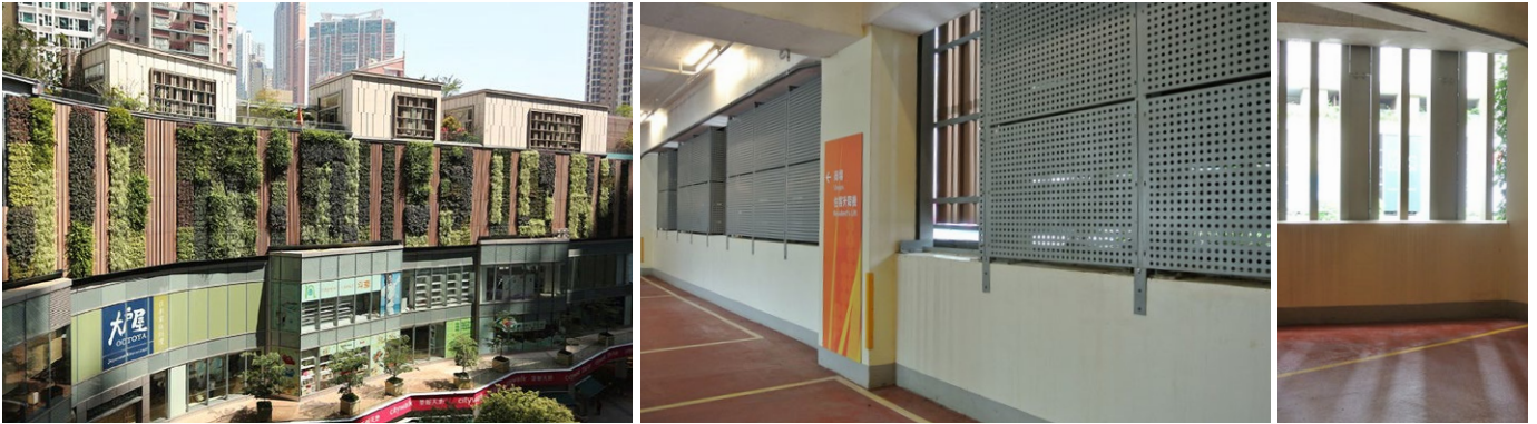
Figure 49 Green wall design as a carpark façade of a shopping mall, Citywalk, Tsuen Wan (Source: Sino Group)
