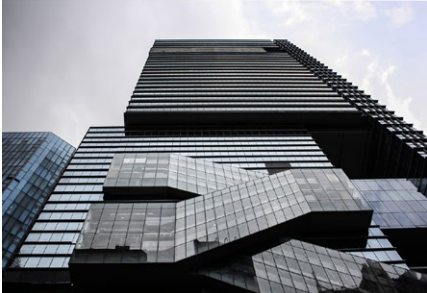
Figure 16 Hysan Place, BEAM Plus V1.1 New building project – platinum rating
