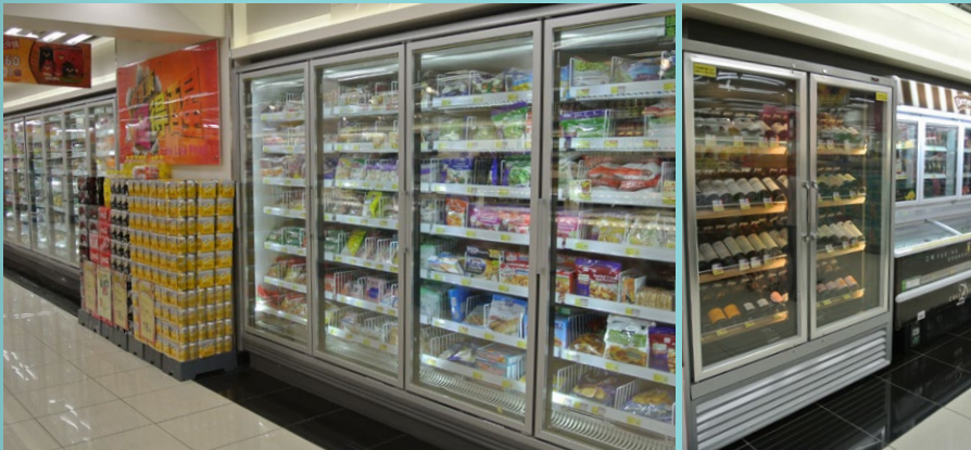
Figure 168 Refrigerators with doors, Wellcome at Causeway Bay
