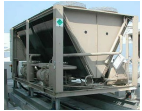
Figure 104 Air cooled chiller
