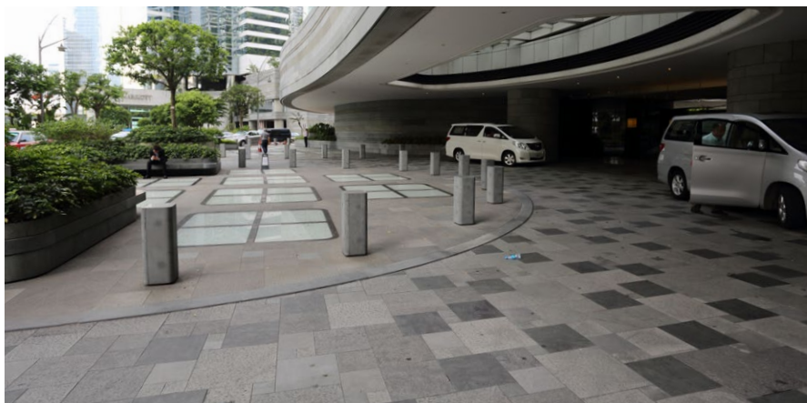
Figure 153 Loading and unloading bay and skylights at Pacific Place, Admiralty
