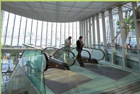
Figure 86 North facing skylight and shading devices in ifc mall, Central
