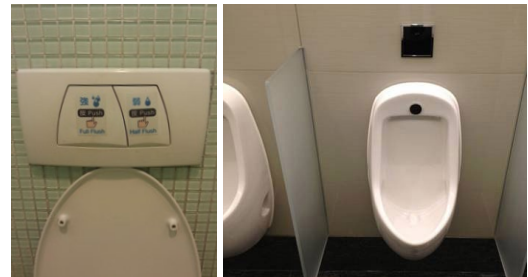
Figure 108 Dual flush & low volume flushing urinal (Source: Kai Shing Management Services Limited)
