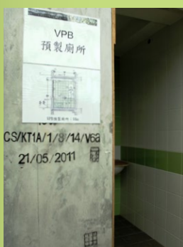
Figure 126 Precast volumetric bathroom (Source: BEAM Society Limited)
