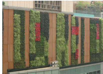
Figure 72 Green wall in Citywalk, Tsuen Wan (Source: Sino Group)
