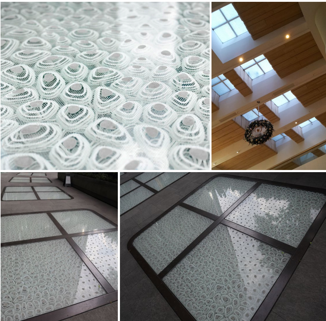
Figure 83 Fritted glass pattern of the skylights at Pacific Place, Admiralty (Source: Swire Properties Limited)
