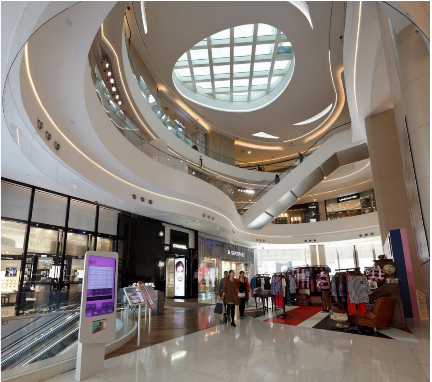
Figure 32 Use of daylight at Hysan Place, BEAM Plus V1.1 new building project – platinum rating
