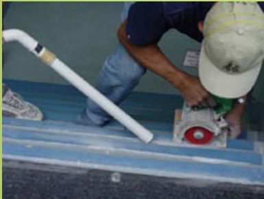
Figure 135 Use of vacuum cleaner to reduce dust impact (Source: Environmental Protection Department)
