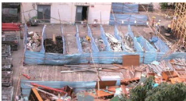
Figure 121 On-site waste sorting facilities for recycling and reuse (Source: Environmental Protection Department)
