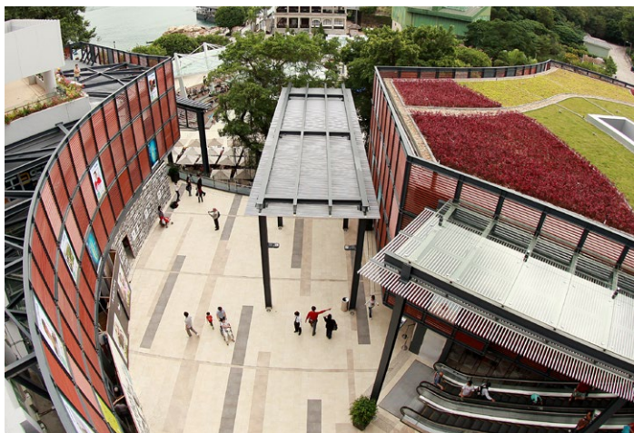
Figure 4 Stanley Plaza, BEAM 4/04 new building project – platinum rating (Source: The Link Management Limited)
