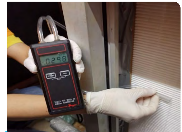
After installing EcoSonic
