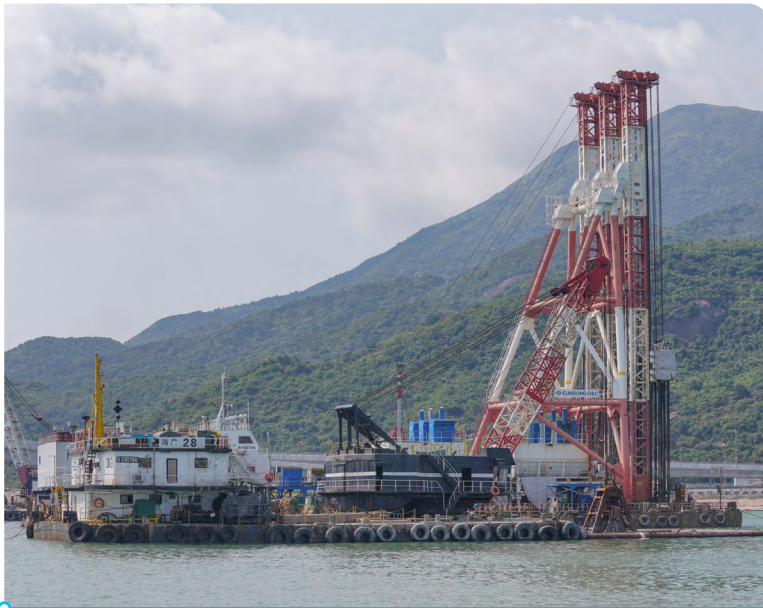
Deep Cement Mixing barge
