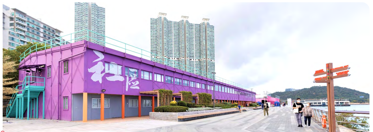
Building Façade next to East Entrance
