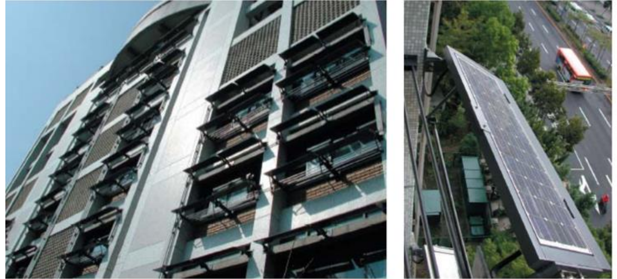
Installation of outer sun-shading incorporating with solar cell system
