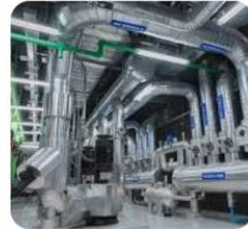
Chilled Water Piping
